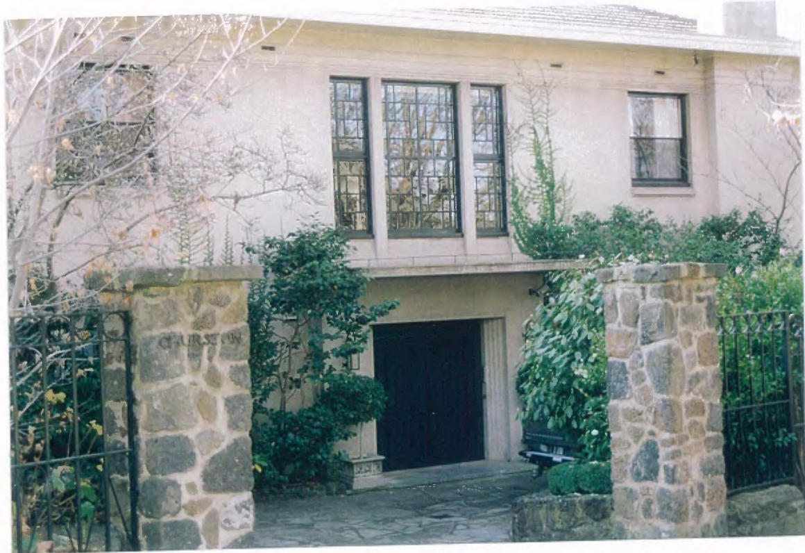
1 Main entrance and gateway with patterned glazing bars, a characteristic of Martin stairwells
