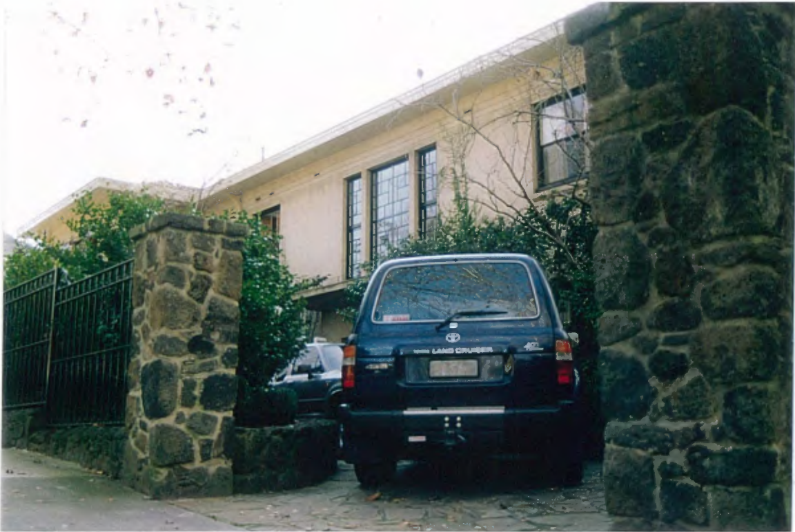
3 East driveway entry with stair well windows and gateway, refer early photographs
