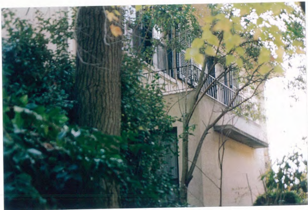
6 Detail of side balcony 5 Linlithgow Road, Toorak
