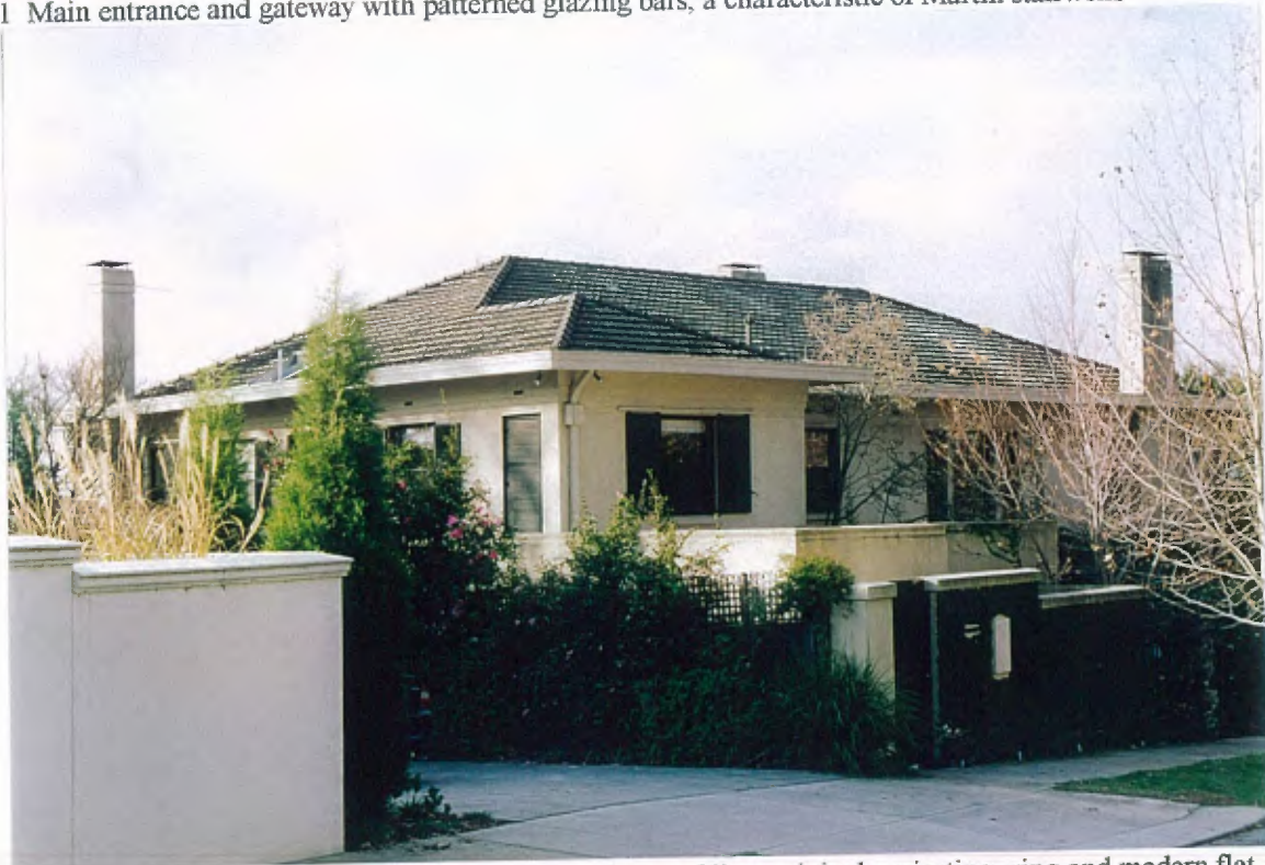
2 Overall view from south west, showing low pitched roof line, original projecting wing and modern flat roofed projection
