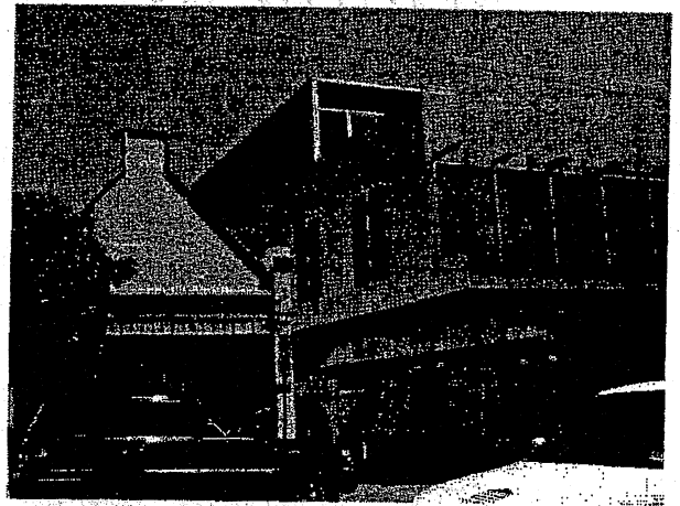
Early 20th century (no 416) and modern building adjacent (414)
