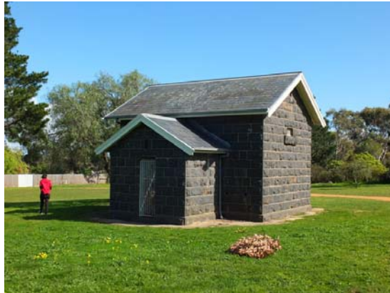
Former Lock Up, Bannockburn
