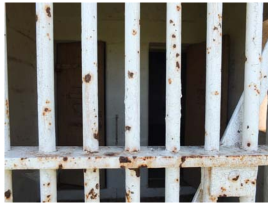
Interior of lock up porch looking to the cells at the rear.
