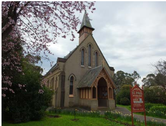
St. Paul's Anglican Church, Inverleigh, 2012.
