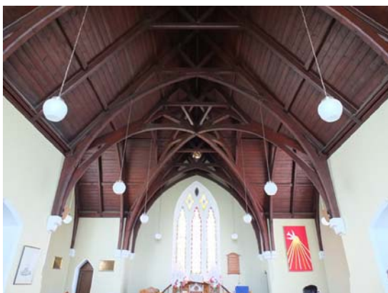
Church interior, roof detail.
