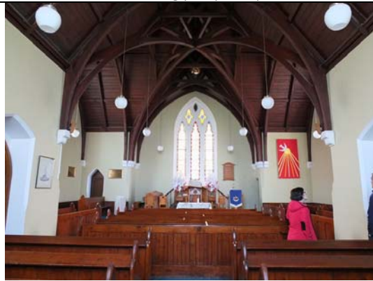
Church interior, looking north towards chancel.
