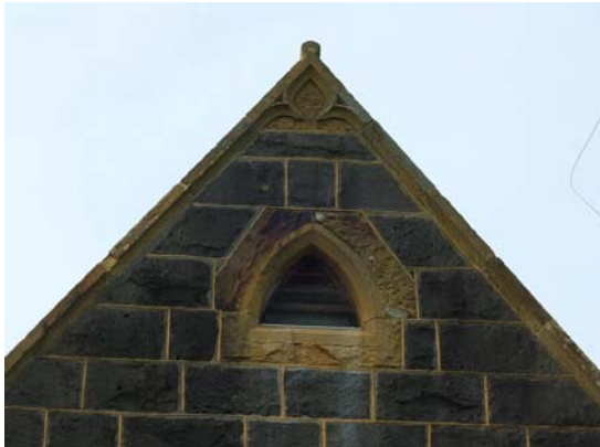
Detail of gable end showing Italian-pointed ventilator and stylised half-trefoil motif near the apex.
