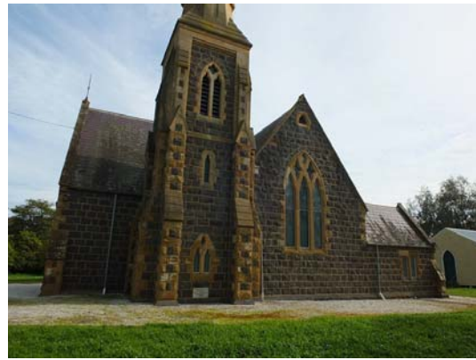
Rokewood Presbyterian Church, side (east) elevation showing detailing of tower (the light stone below the ground floor windows is the memorial stone).
