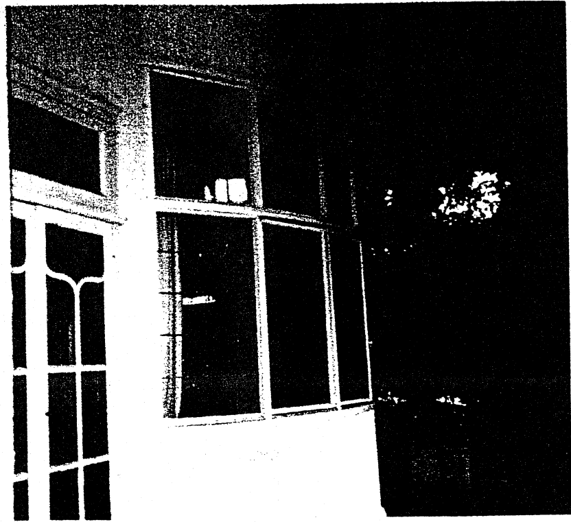
Figure 13 Corner bow window and French doors to sitting room
