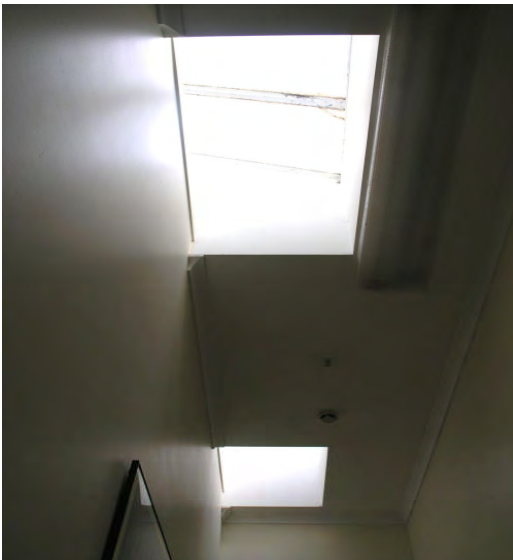
Photograph 9: Ceiling windows visible from central hallway Source: HLCD, 22.05.07
