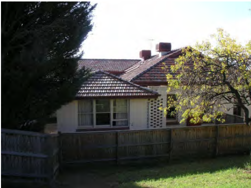
Photograph 3: South west elevation showing later extension to B1 Source: HLCD, 22.05.07
