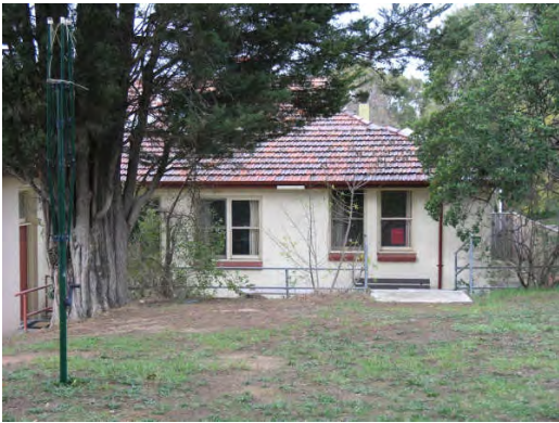
Photograph 5: North west elevation of B1 Source: HLCD, 22.05.07
