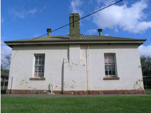
Photograph 10: North east elevation of B3 façade Source: HLCD, 22.05.07
