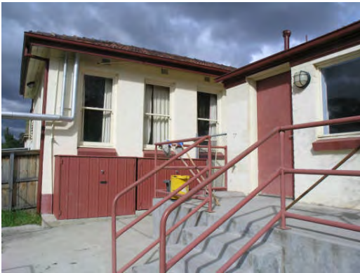
Photograph 8: North east elevation of B1 showing rear additions Source: HLCD, 22.05.07
