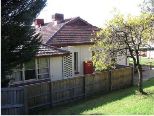
Photograph 4: View showing roofline of original section of B1
