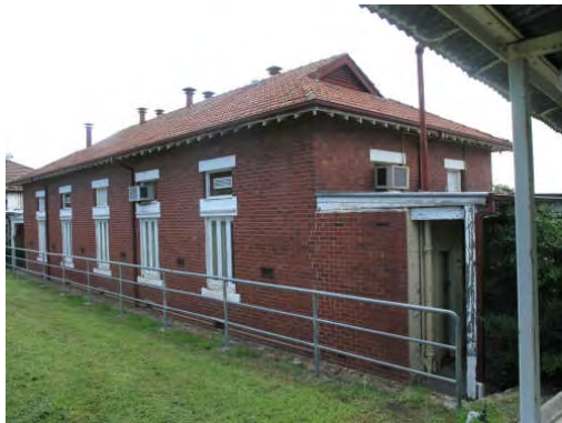
Photograph 23: South west elevation taken from south eastern view showing change in building form with the addition of two skillion toilet blocks Source: HLCD, 22.05.07
