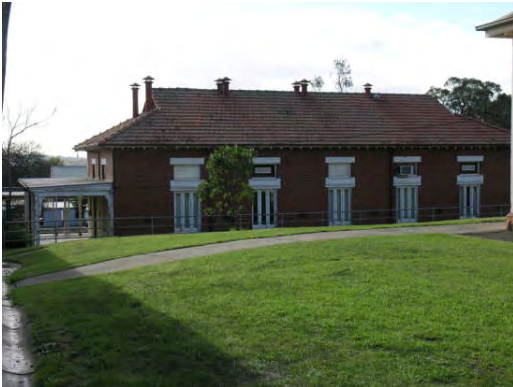
Photograph 22: South west elevation of B6 Source: HLCD, 22.05.07
