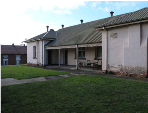
Photograph 11: North west elevation of B3 Source: HLCD, 22.05.07
