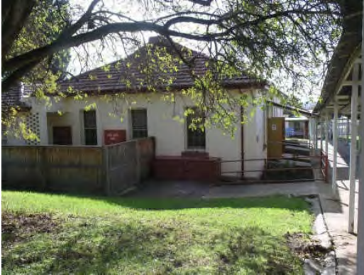
Photograph 2: South west elevation of original section of B1 Source: HLCD, 22.05.07
