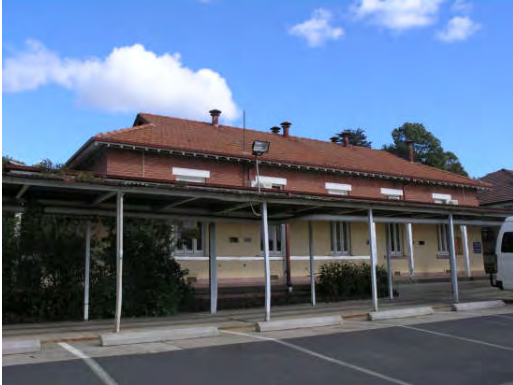
Photograph 21: North east elevation of B6 Source: HLCD, 22.05.07
