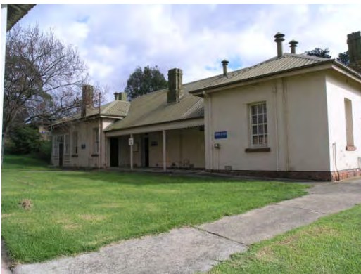
Photograph 12: South east elevation of B3 Source: HLCD, 22.05.07
