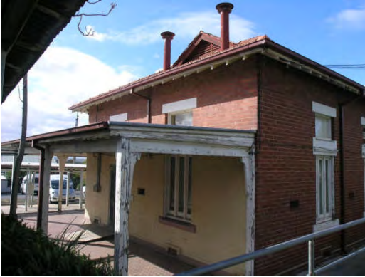
Photograph 24: North west elevation of B6 Source: HLCD, 22.05.07
