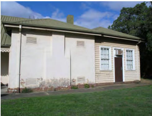
Photograph 14 & 15: North west elevation showing removed chimney stack and later vents on either side of chimney Source: HLCD, 22.05.07
