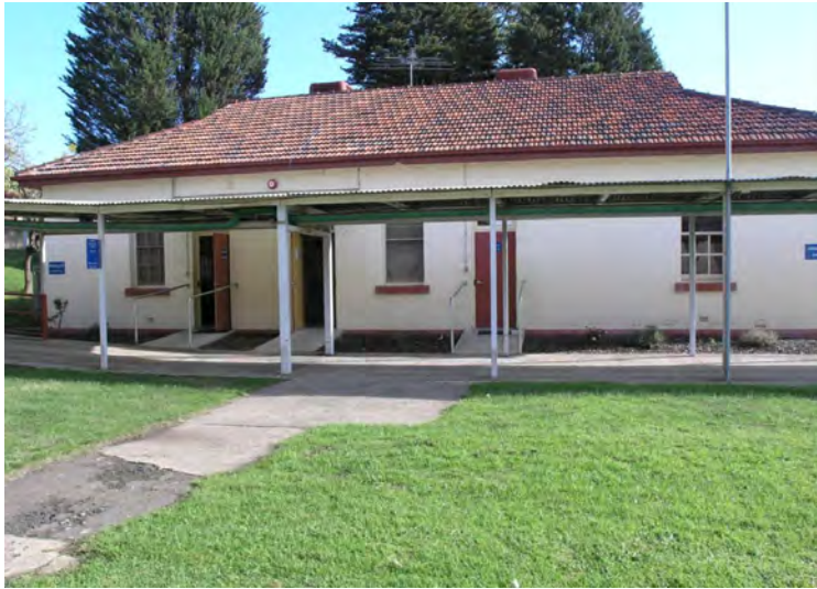
Photograph 1: South east elevation of B1 Source: HLCD, 22.05.07
