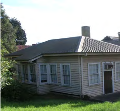
Photograph 13: South west elevation of B3 Source: HLCD, 22.05.07
