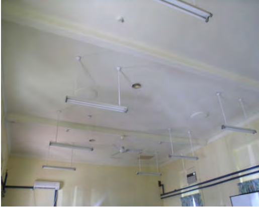
Photograph 27: Ceiling of B6 Source: HLCD, 22.05.07
