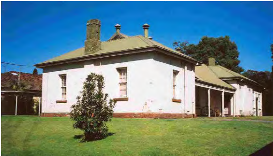
Photograph 38: View taken from the retaining wall south of B6 showing the space surrounding B3. Source: HLCD, 07.08.07
