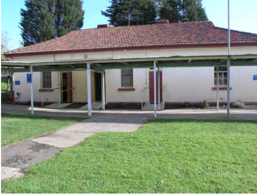
Photograph 1: South east elevation of B1 Source: HLCD, 22.05.07
