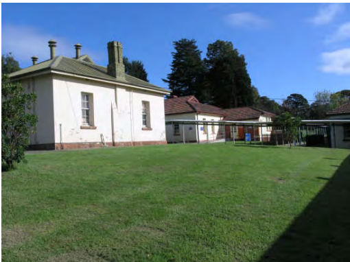
Photograph 35: View of open space between B6, B3 and B1.
