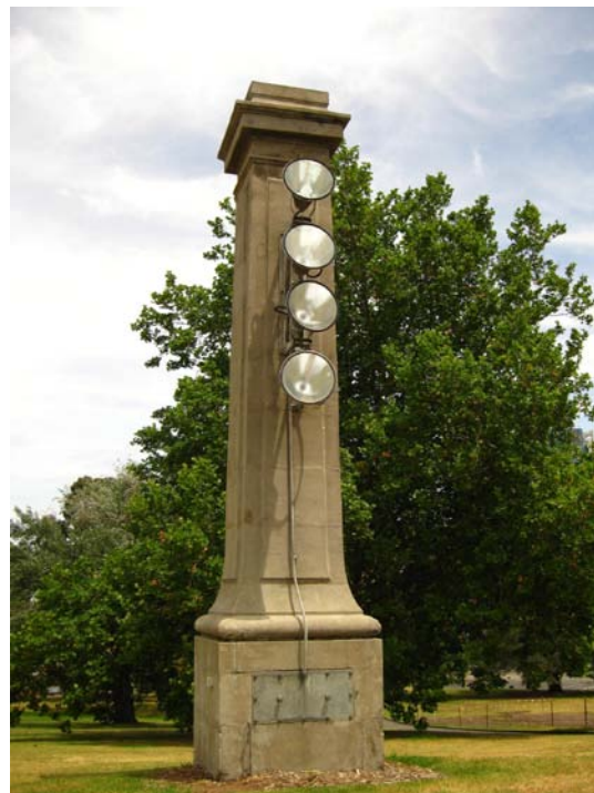
Figure 108 View of the light pylon located to the south-west of the Shrine. Four such light pylons were built around the Shrine as part of the original construction works.
