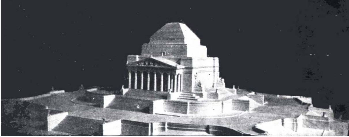
Figure 7 Sculptor Paul Montford produced a model of Hudson and Wardrop's original competition entry design. The shallower roof form and granite walls to the lower terrace can be seen. Source: Building magazine
