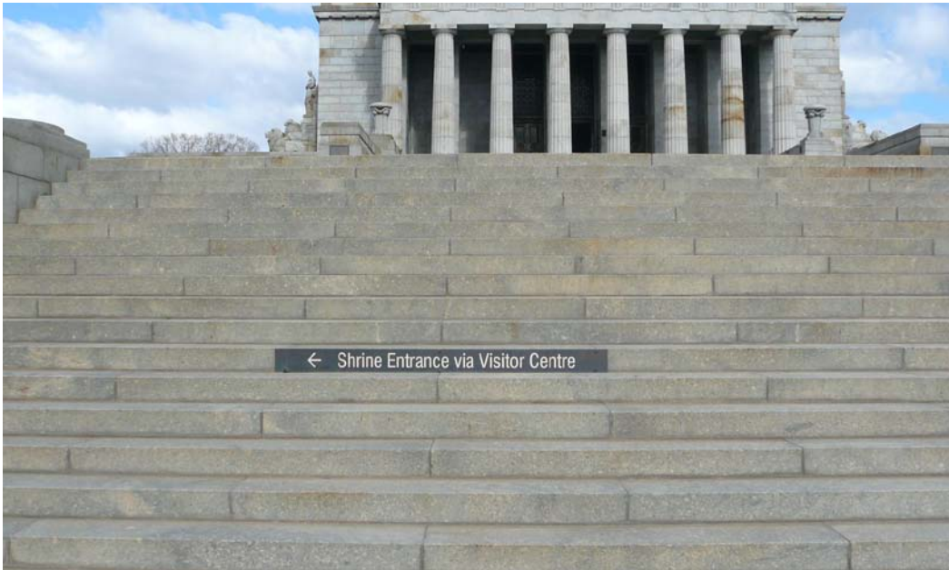
Figure 25 Directional signage to the Visitor Centre fixed to the steps located beneath the northern portion of the lower terrace.
