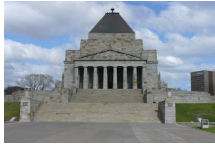
Figure 168 View of the north elevation to the Shrine from the north-south axis to the WWII forecourt.
