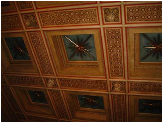
Figure 51 View of the crypt ceiling. Note the finely detailed moulded decoration including a stylised Greek star motif in each central panel.
