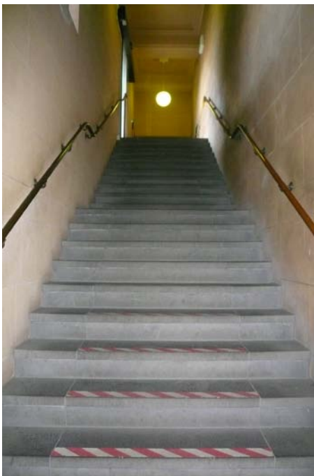
Figure 65 View of the eastern stairs located along the southern side.
