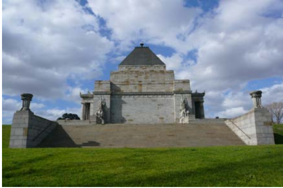
Figure 39 View of the west elevation. Taken from the embankment located below the steps to the lower terrace (western side).
