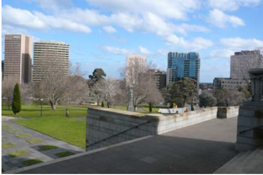
Figure 31 View of the southern portion of the upper terrace (looking southwest). Note the granite retaining wall (centre right of picture).
