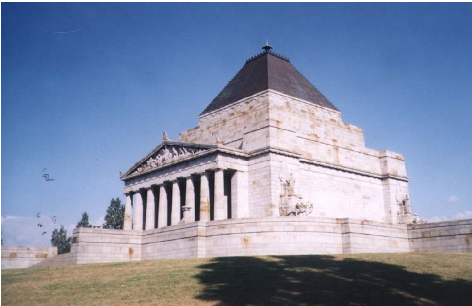
Figure 23 View of the northern and western elevations of the Shrine in 2001. Note that the only major external alteration to the Shrine at this point was the copper sheeting to the dome, which had been carried out by the early 1970s to counter water penetration.
