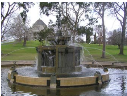
Figure 103 View of the fountain located in the south-western corner of the Reserve site. Note that this element was designed by Hudson and Wardrop, the original Shrine architects.
