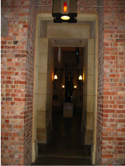
Figure 56 View of the new opening located between the northern side of the undercroft and the crypt passage.
