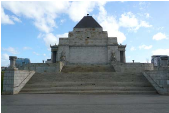
Figure 40 View of the east elevation Taken from the area in front of the Garden of Appreciation (looking east).
