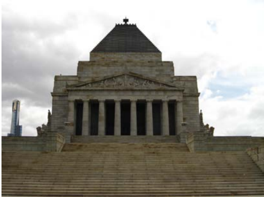
Figure 35 View of the principal south elevation taken from the lower terrace.
