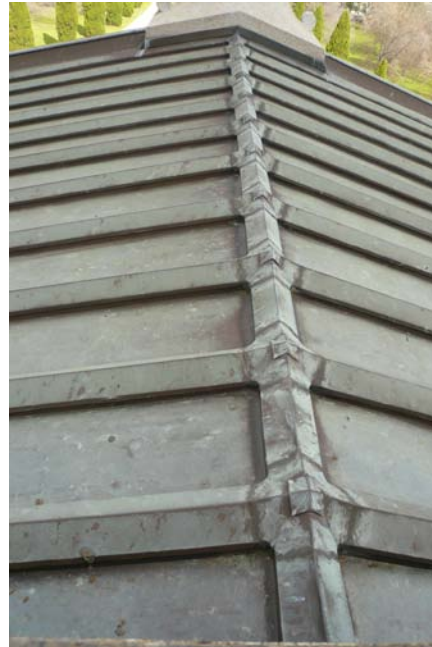
Figure 47 View of the roof to the southern entrance portico.
