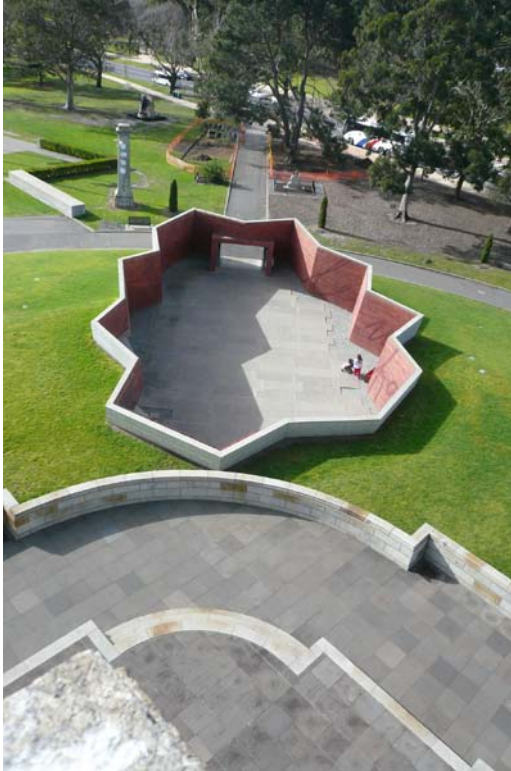
Figure 74 View of the entrance courtyard to the Visitor Centre. Taken from the north-east corner of the lower balcony to the Shrine.
