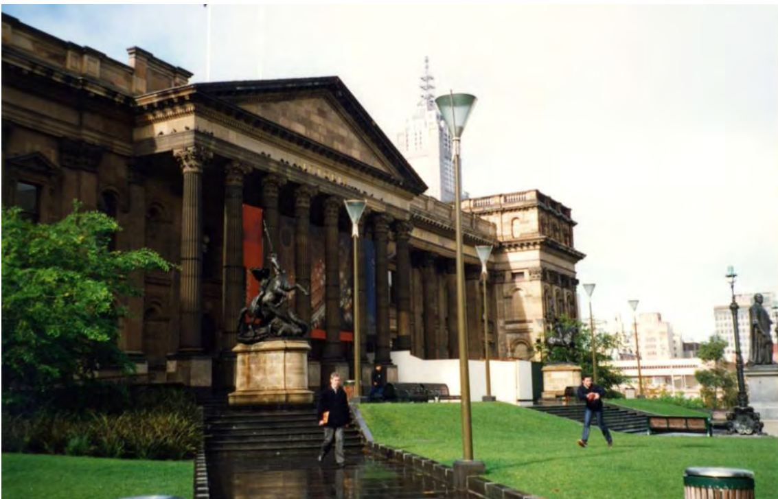
Figure 43 Another view of the refurbished forecourt, from the north-west (2008).
