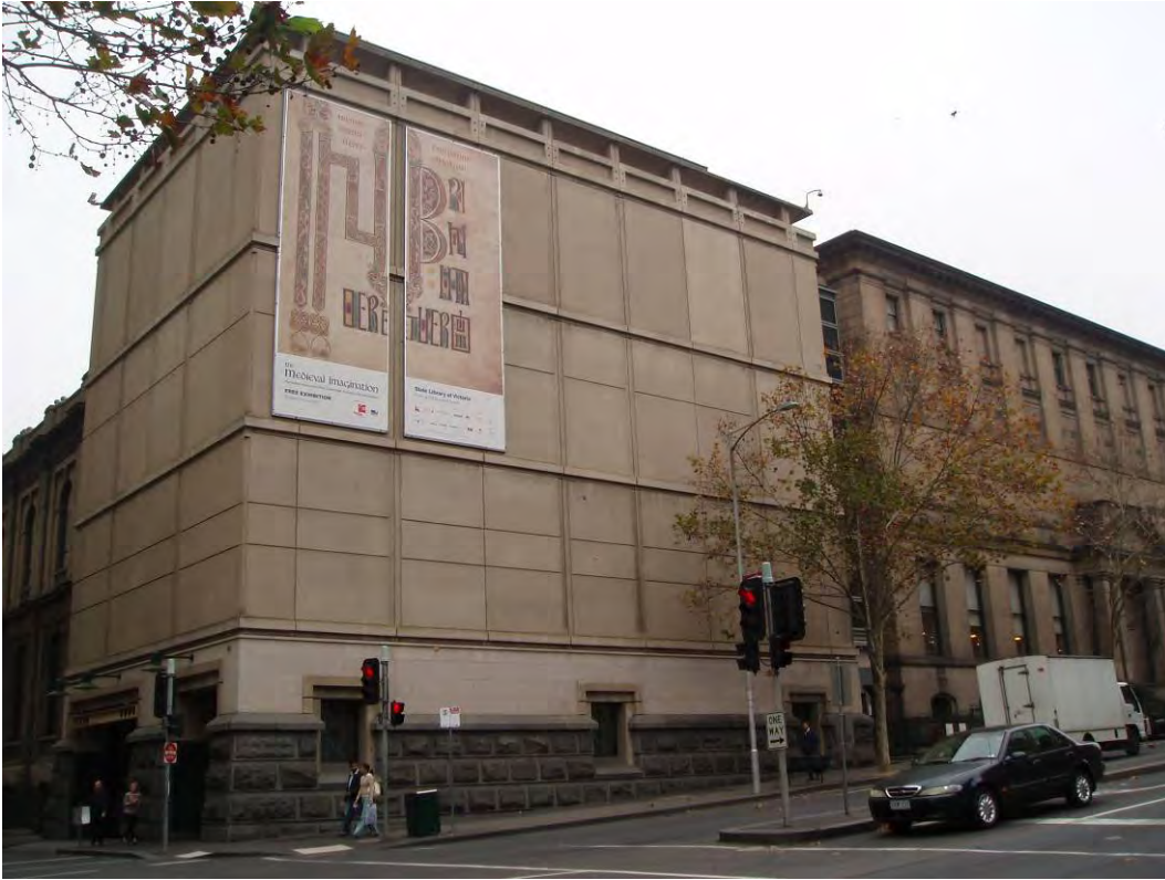
Figure 65 Building Q, the South East Wing.
