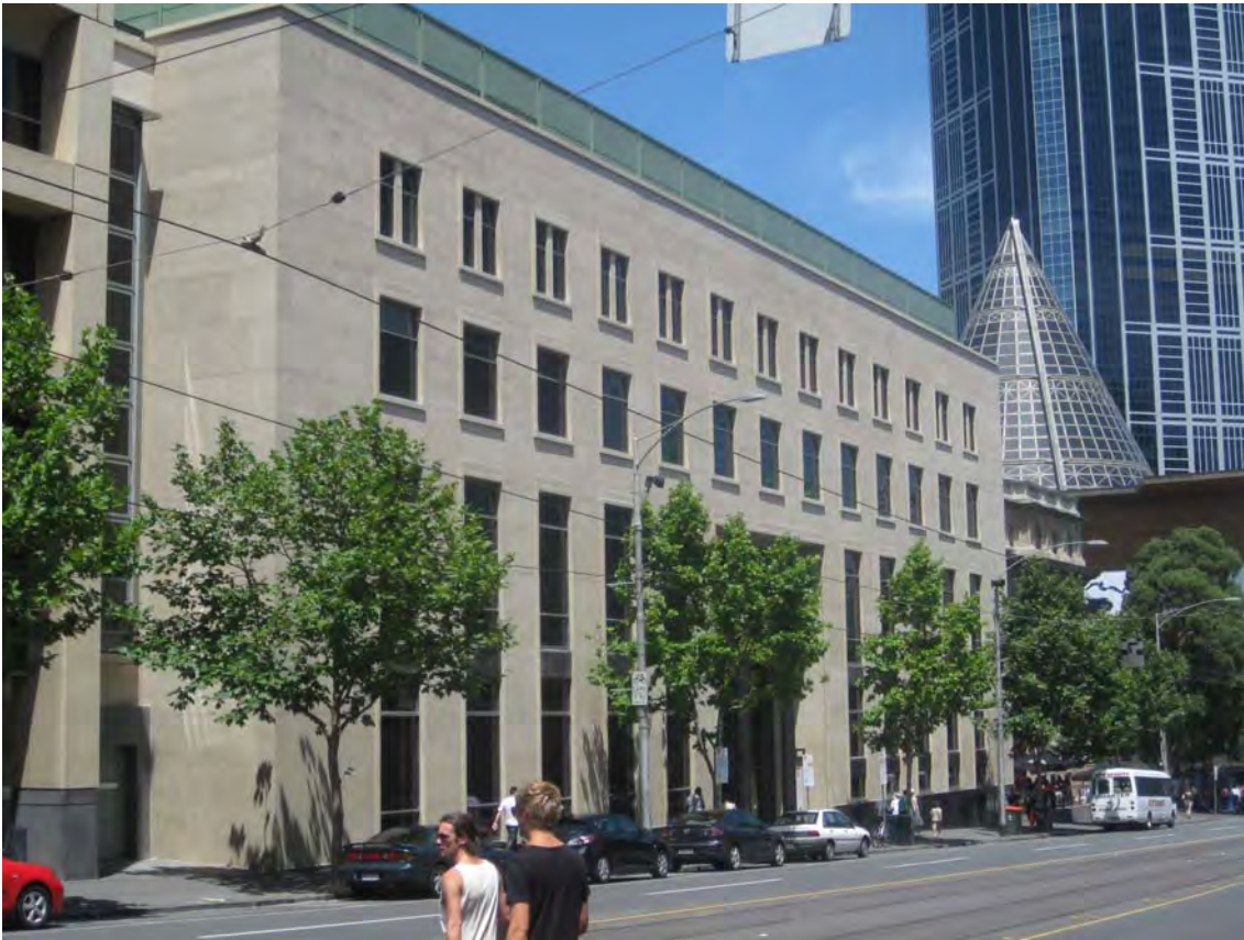
Figure 64 The former La Trobe Library, 2011 (completed 1965).
