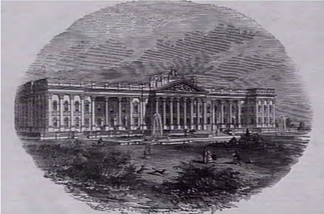
Figure 25 Samuel Calvert's view of the building – the earliest identified - is thought to date from 1859.
