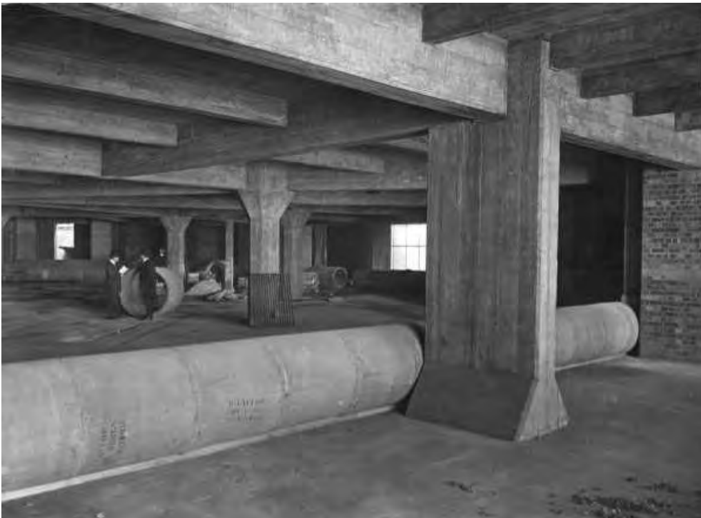
Figure 12 Air circulation services being installed in the Library basement, c. 1913.
