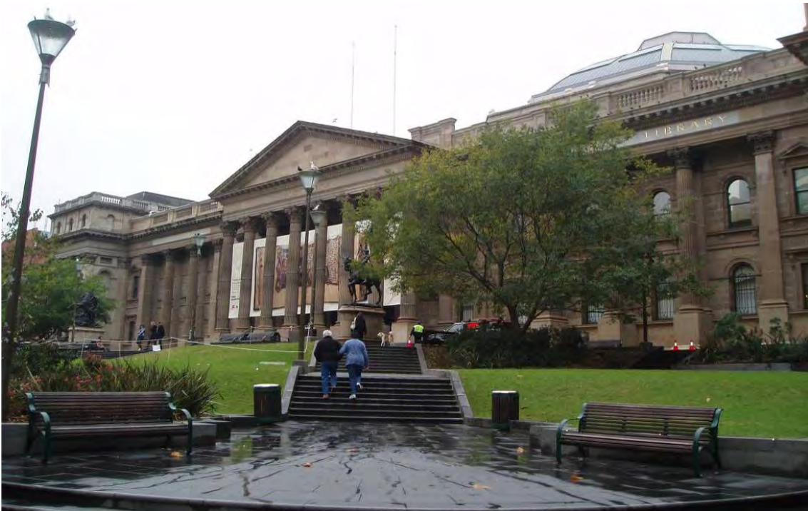
Figure 42 Recent view of the forecourt from the south-west (2008).
