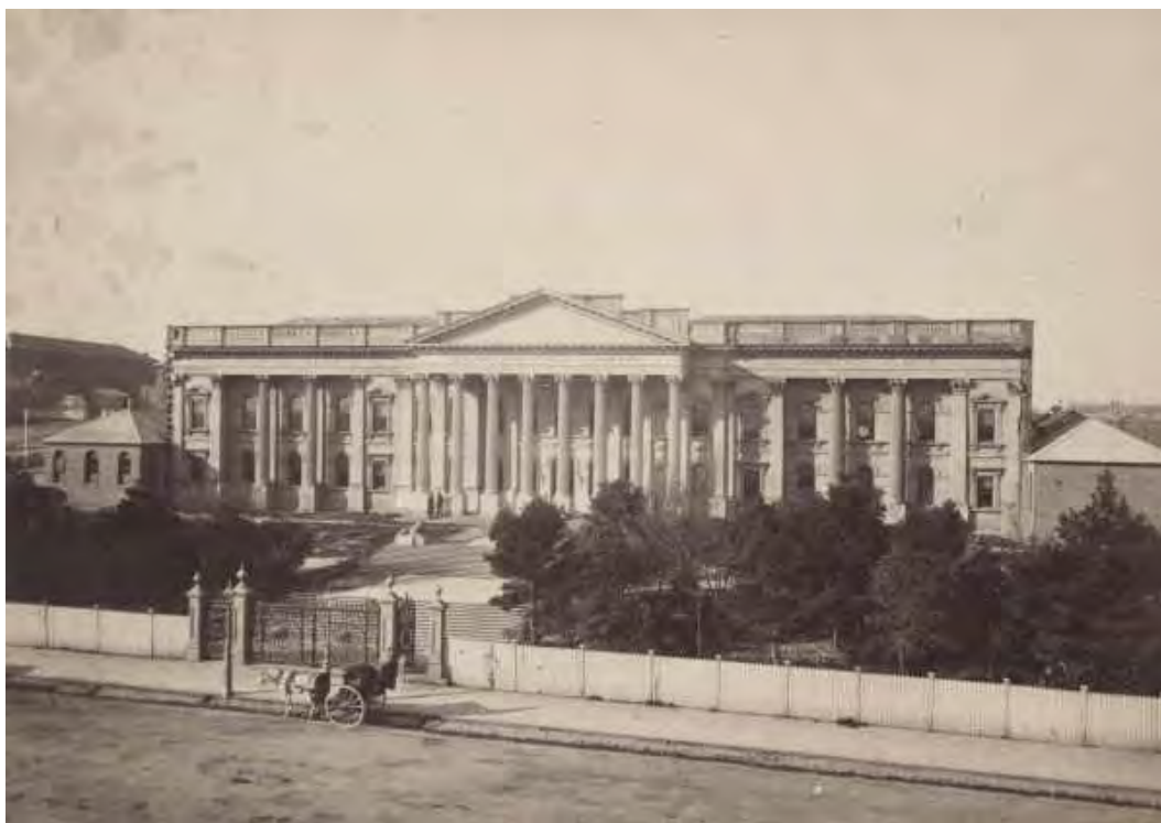
Figure 6 The exterior of the State Library building, after the completion of the portico, c. 1873. Note the new wrought iron entrance gates.
