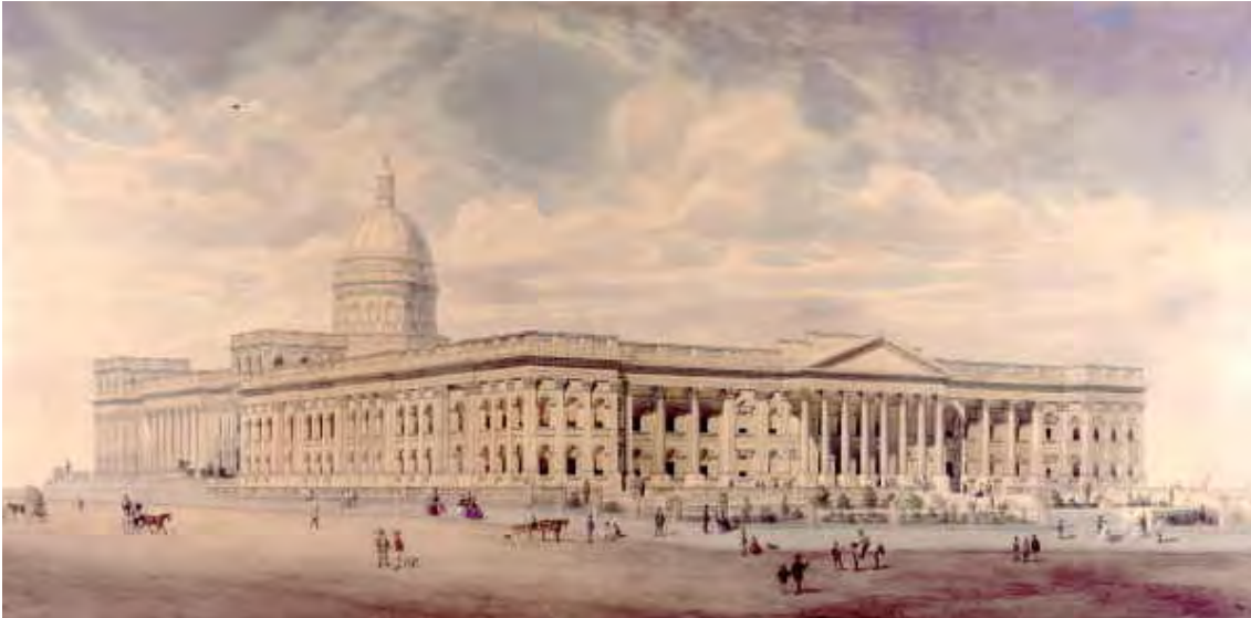
Figure 30 Master Plan, 1860: 'The Public Library', 1860, as depicted by Nicholas Chevalier. Source: Pictures Collection, State Library of Victoria.
