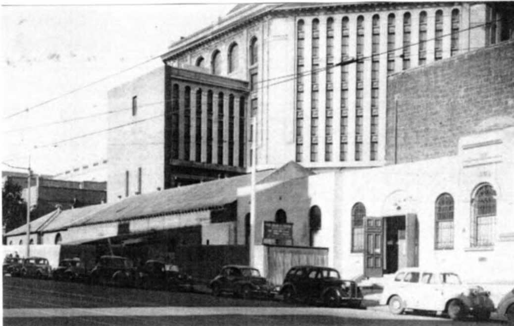
Figure 39 The La Trobe Street buildings, c. 1939-45: View from La Trobe Street, c. 1945. Source: Pictures Collection, State Library of Victoria.
