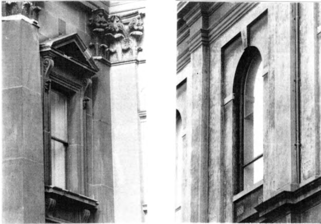
Figure 36 Window detailing to the Swanston Street façade (1859) on left and the Little Lonsdale Street façade (1886) on the right.
