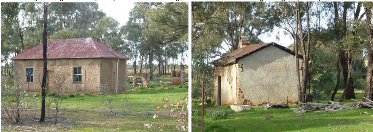
Left: West and south elevation of the cottage, note ruins of former kitchen at rear. Right: The outbuilding as viewed from Caldow Road. Note poor condition of the roof and render.
