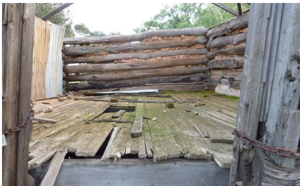
June 2010 – Left: Raised floor and remnant mud and brick pugging to the eastern store. Right: View of site from north-west, with the former dwelling at left.
