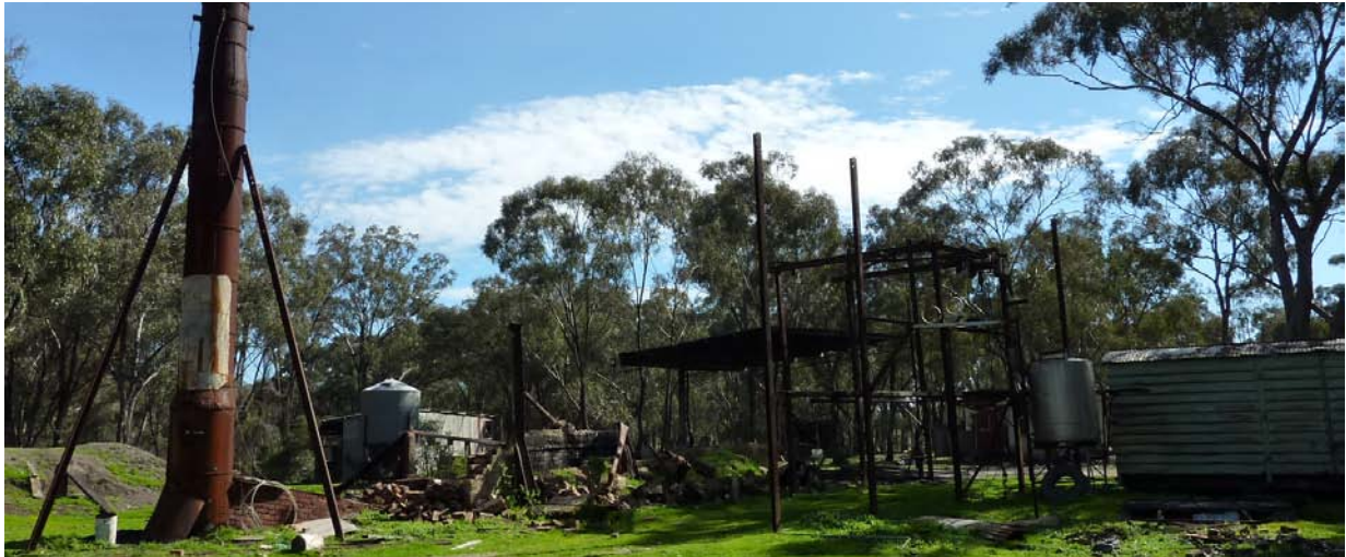
From left, looking north: Metal stack; remnants of brick boiler housing; gantry for truck-mounted vat; and rail carriage (former eucalyptus cutter's hut).
