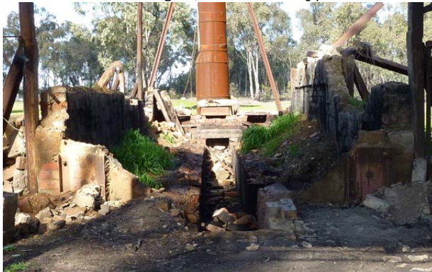
Left: Brick housing for boiler, removed 2010. Right: In-ground brick vat.
