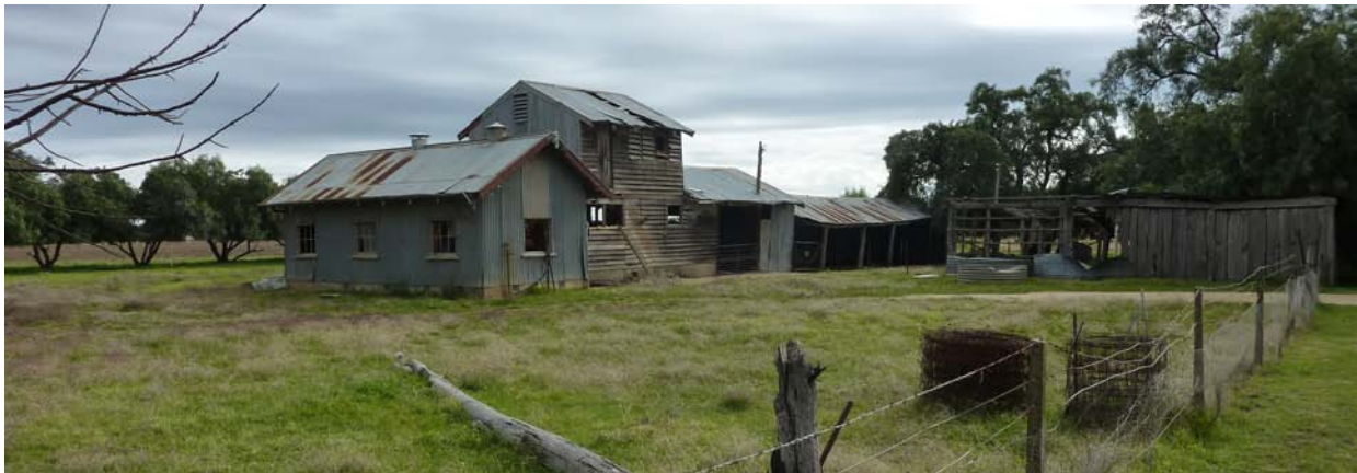
McKenzie's Tomato Seed Extraction Factory looking east.
