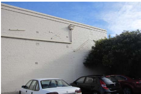
Left: East elevation, note angled brick course, evidence of a pre-existing structure in this location. Right: Aerial view, 2010 (Source: City of Greater Bendigo).
