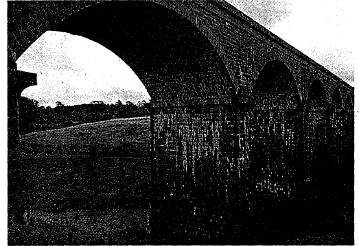
Railway Bridge over Coliban River, Malmsbury
