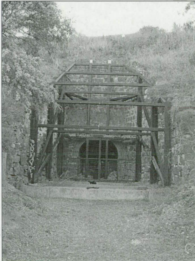
Limeburners Point Lime Kiln (Brad Duncan Collection)
