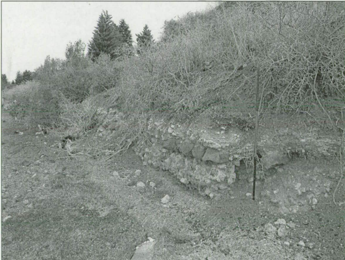
Limeburners Point Structure Pad Site
