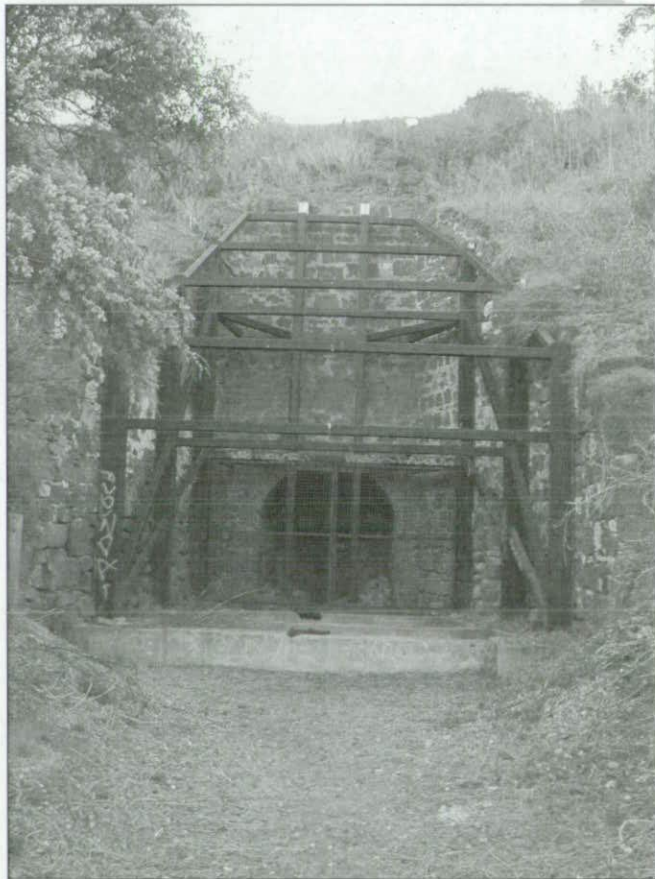
Limeburners Point Lime Kiln (Brad Duncan Collection)
