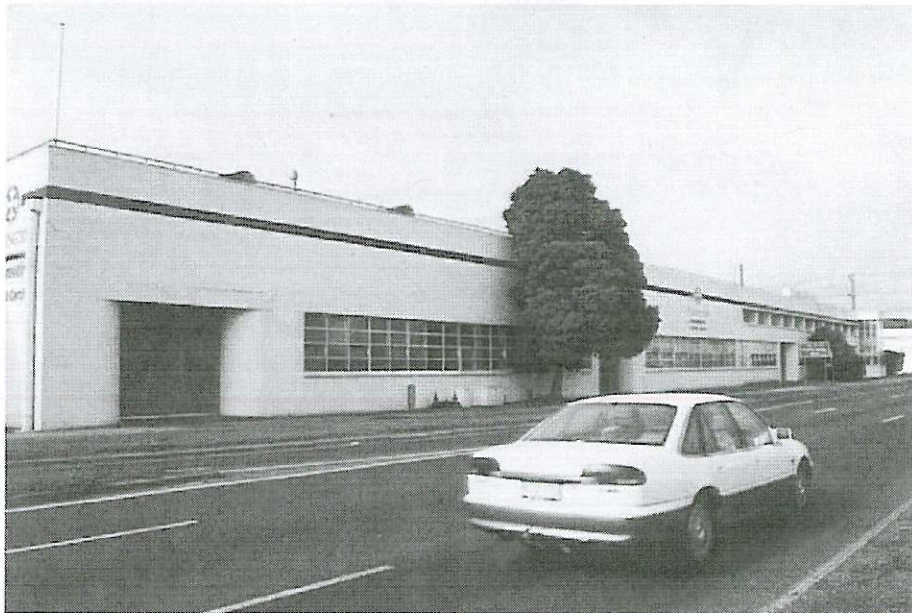
View of the West elevation (looking south) recommended for protection on the planning scheme.
