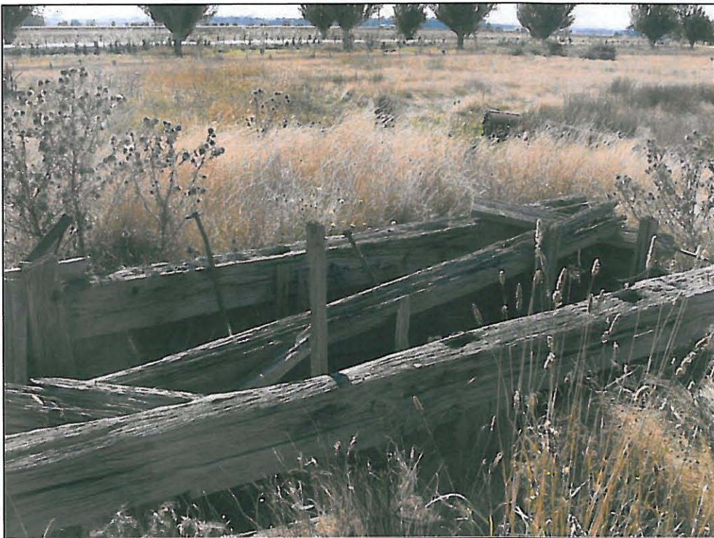
Fig. 7: View of mine shaft to the south, facing northeast (W. Anderson, 8/4/2011)
