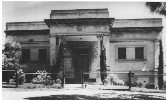
Figure 12 Sorrento Masonic Lodge, Point Nepean Road.
