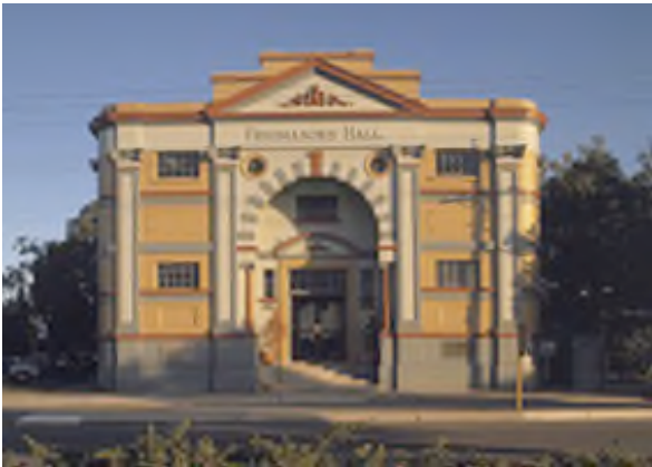
Figure 16 Masonic Hall, Subiaco
