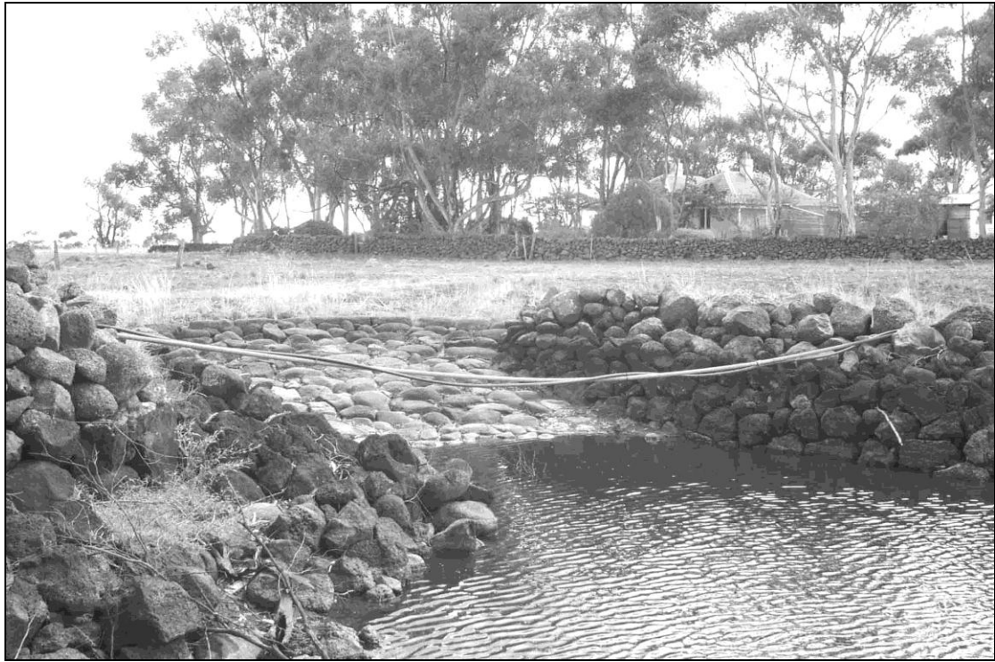
Part of the dry stone wall dam, with cobbled ramp, in front of homestead.
