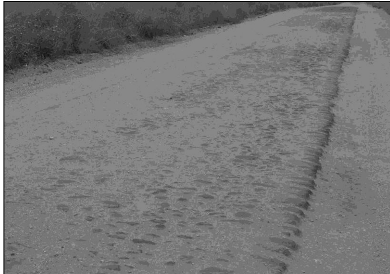
Gourlay Road (Place No.366)
