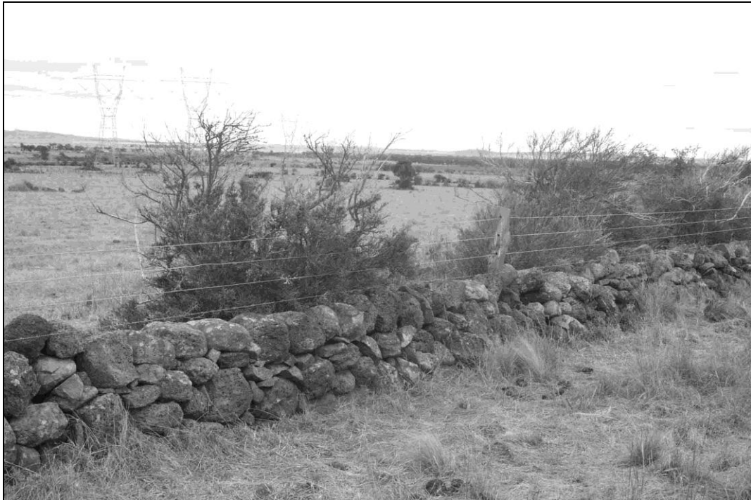
Drystone wall in good condition on the north boundary of the Moloney property.
