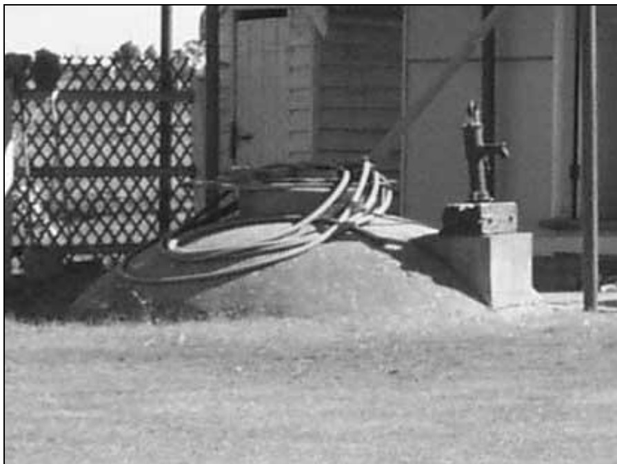
Domed cement rendered brick underground tank, with iron handpump.
