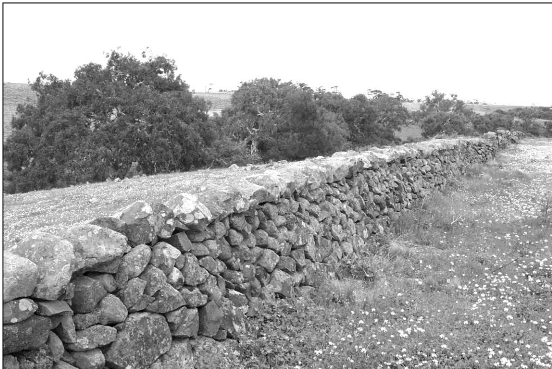
Dry Stone Wall in front of the cottages, overlooking Kororoit Creek. Built late 1860s.
