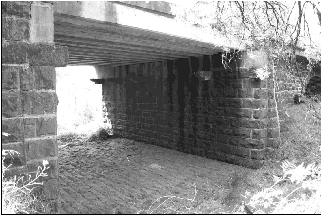
The girder span, showing the shaped bluestone corbels, bluestone paved bed. Concrete girders have replaced the original timber ones. The round arch span is adjacent.
