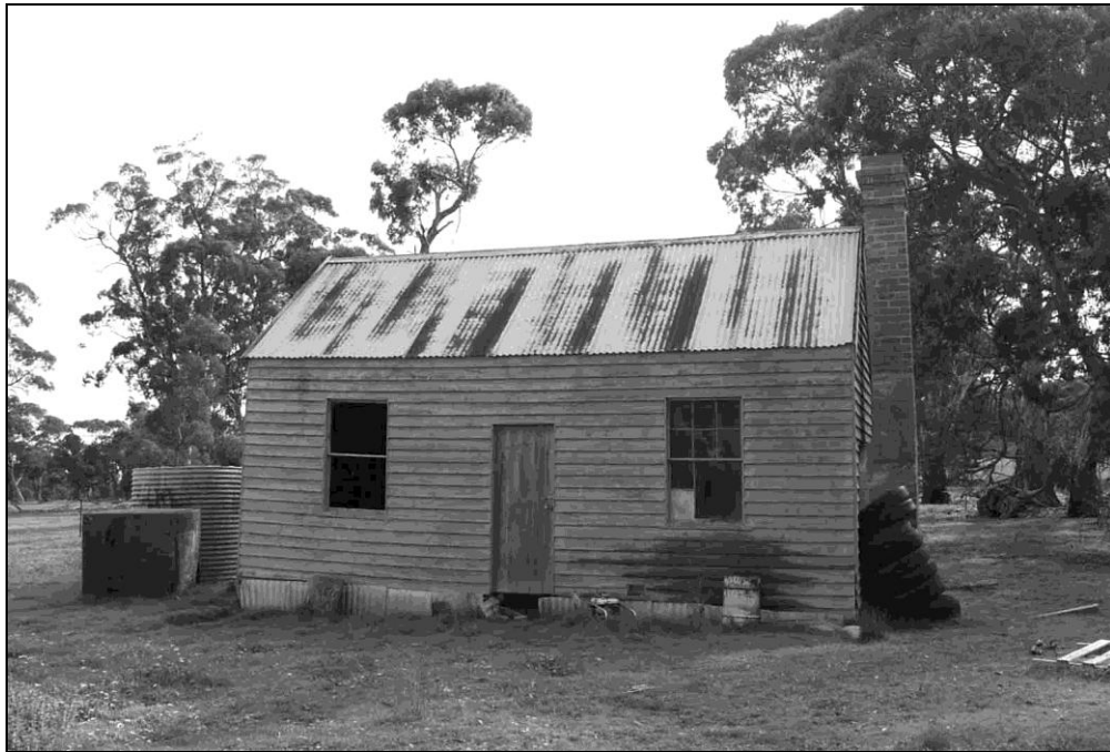
Workers' (probably shearers') quarters behind shearing shed.
