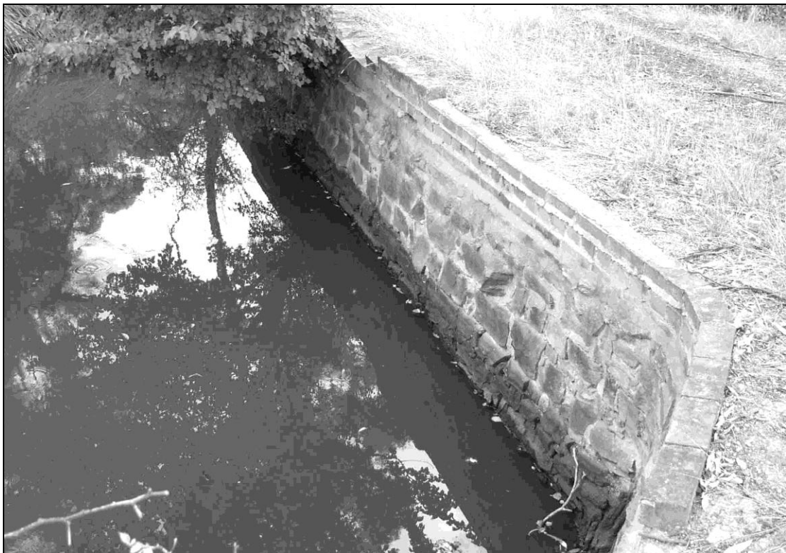
The finely constructed dam wall.
