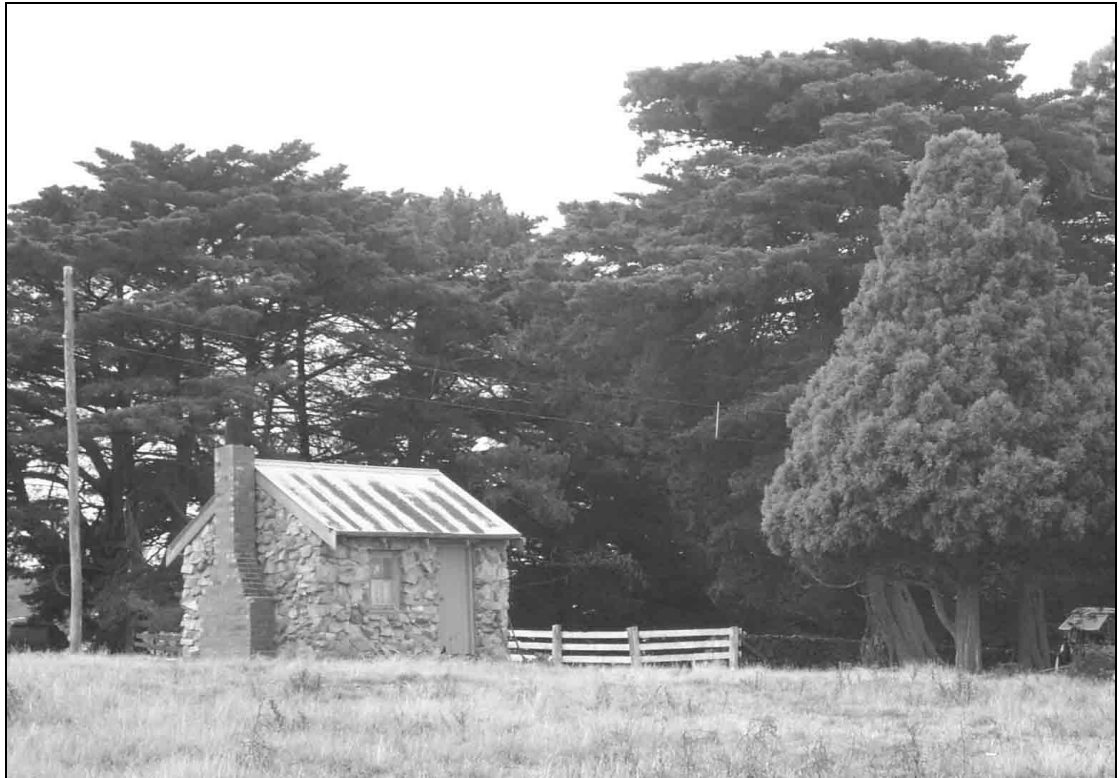
c.1944 Italian POW-built cottage and a Bhutan cypress.
