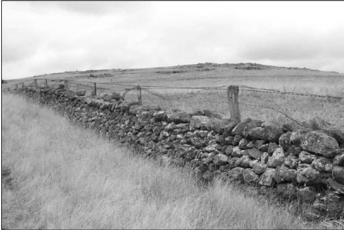
Dry Stone Wall: cope stones, and remnant of composite post and top-rail fence.
