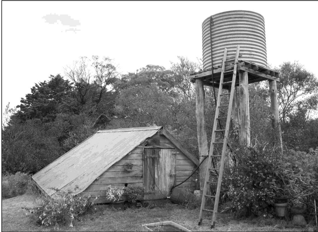
Underground water tank covered with gable roof, and adjacent corrugated steel header tank. The steel header tank was demolished in 2003.
