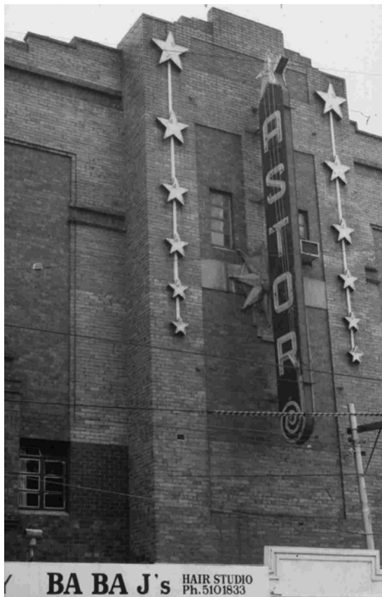
Figure 7 The highly animated Astor Cinema sign of 1936 continues to operate at this popular Art Deco cinema in East St Kilda. The stars on the façade are also outlined in neon. Blade signs similar to the one shown here, are the most numerous survivors of the neon era.
