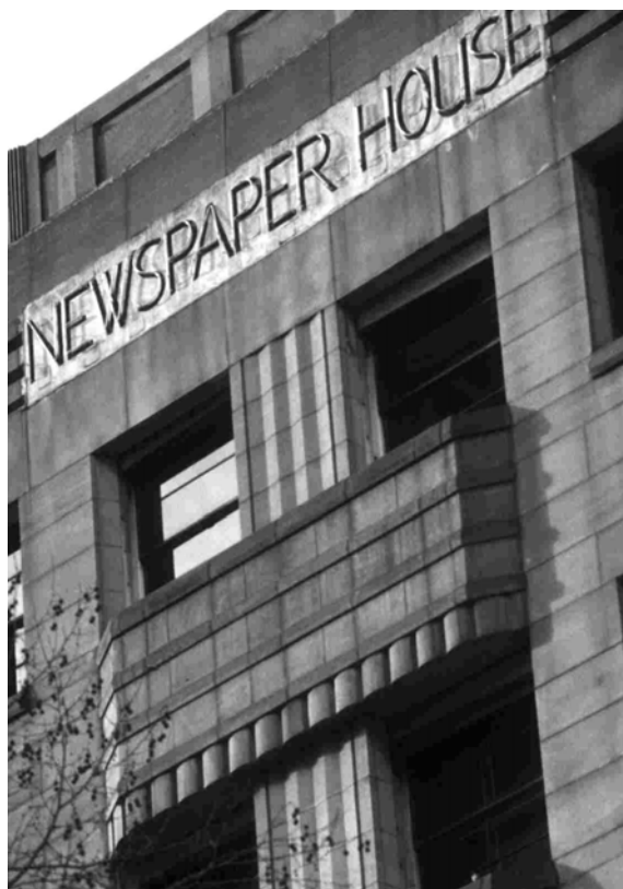
Figure 9 Newspaper House, Collins Street Melbourne. Constructed in 1933, the building incorporated neon signage on a base embedded in the facade. This is possibly the oldest surviving neon in Melbourne and is rare for its architectural integration into the design of the building. The sign no longer operates.
