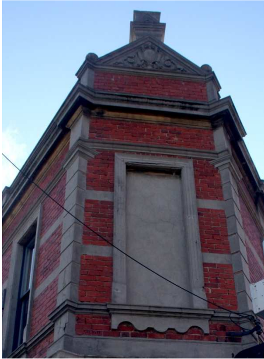
Figure 8 Parapet pediment raised over the corner of the building, with sunflowers and blind window
