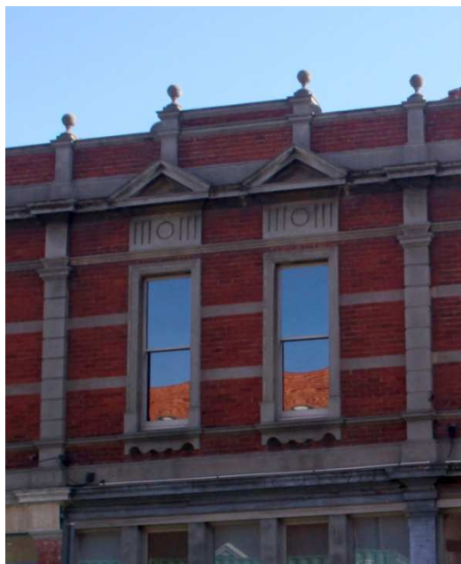
Figure 7 Some of the distinctive Polain detailing used: parapet piers rising from the apices of window pediments
