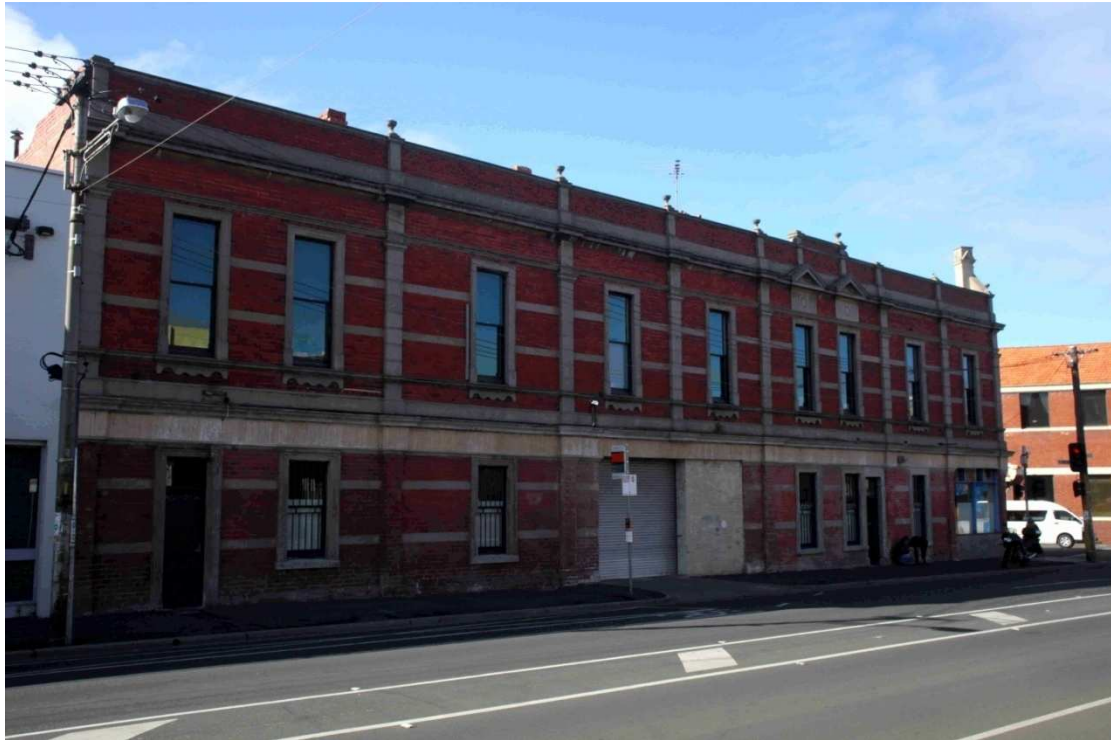
Figure 3 Nicholson Street elevation showing new opening where a shopfront once existed.
