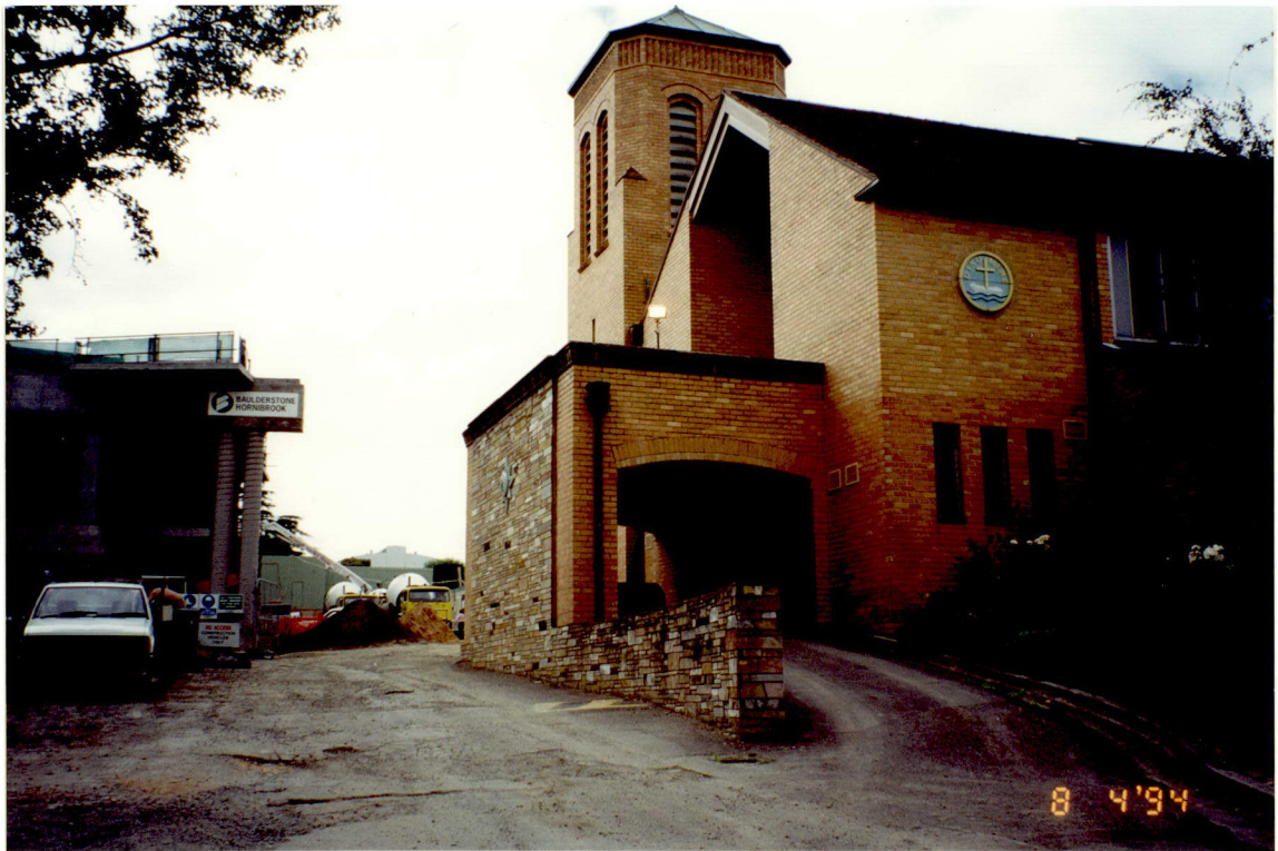
Impact of new music school on main block (graded 'A') & chapel (graded 'B')
