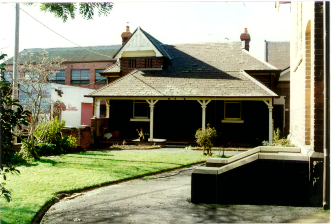
3 Hepburn Street (part of Auburn Uniting Church) complex
