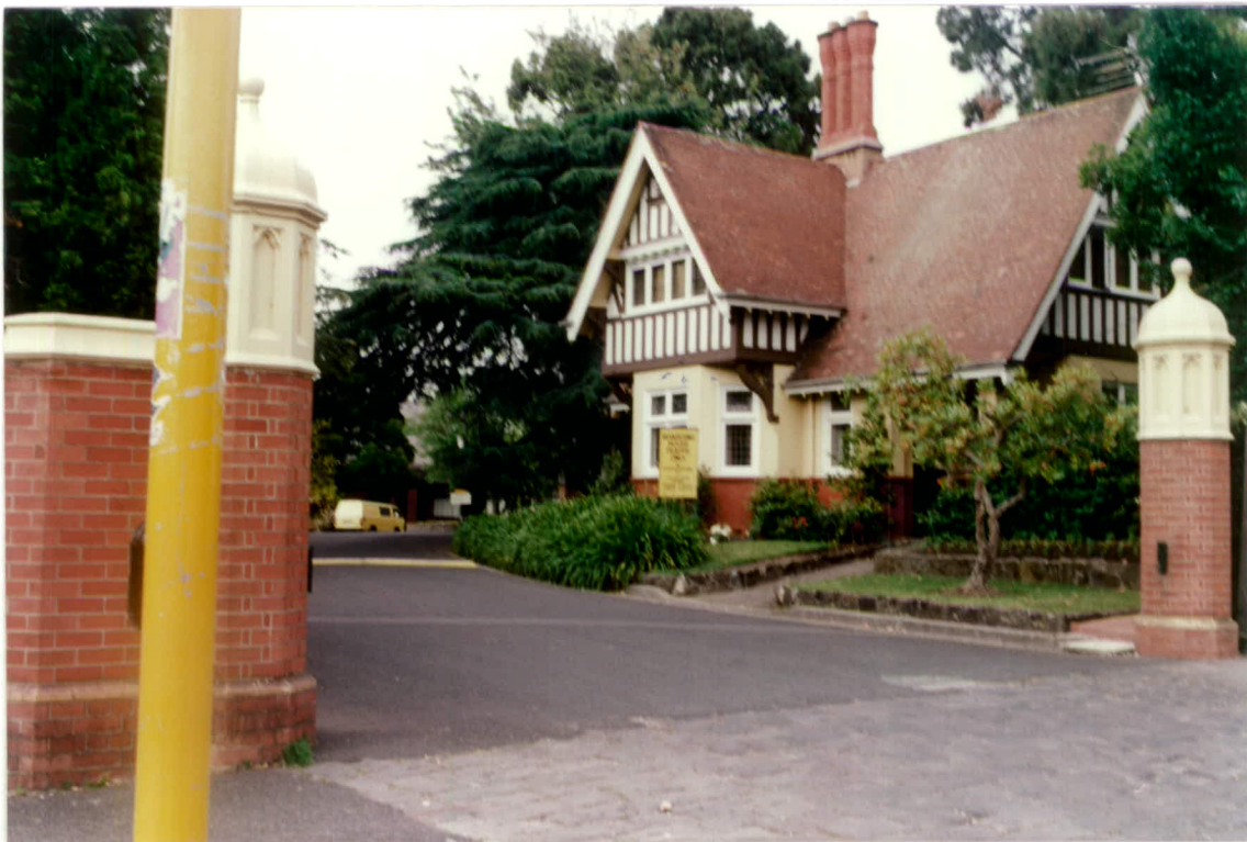
Main Entrance 491 Glenferrie Road Scotch College
