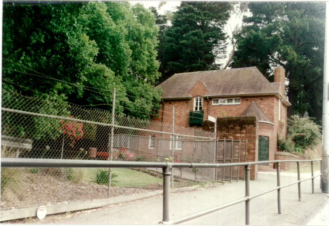
Gatehouse John Monash gates and Lodge
