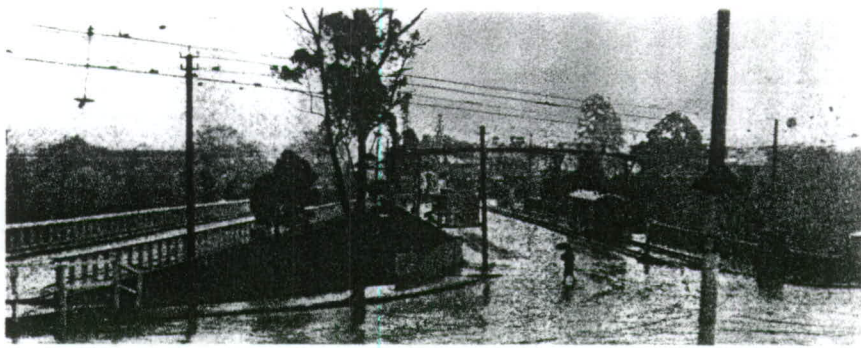
Two Hawthorn bridges: the Board's temporary structure is on the left
