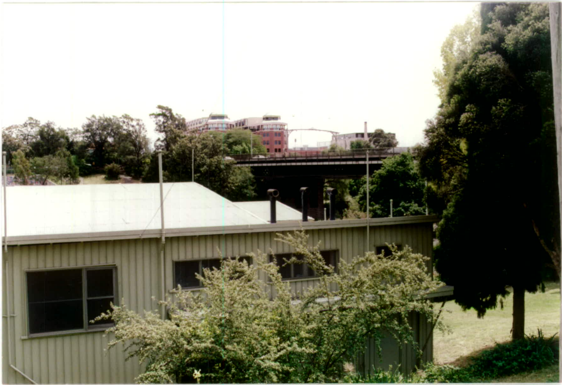
Burwood Road Bridge
