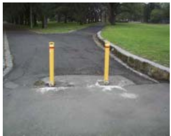
Figure 68 Early cast iron bollards (left) and later steel bollards (right)
