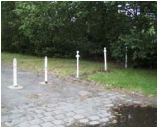
Figure 68 Early cast iron bollards (left) and later steel bollards (right)
