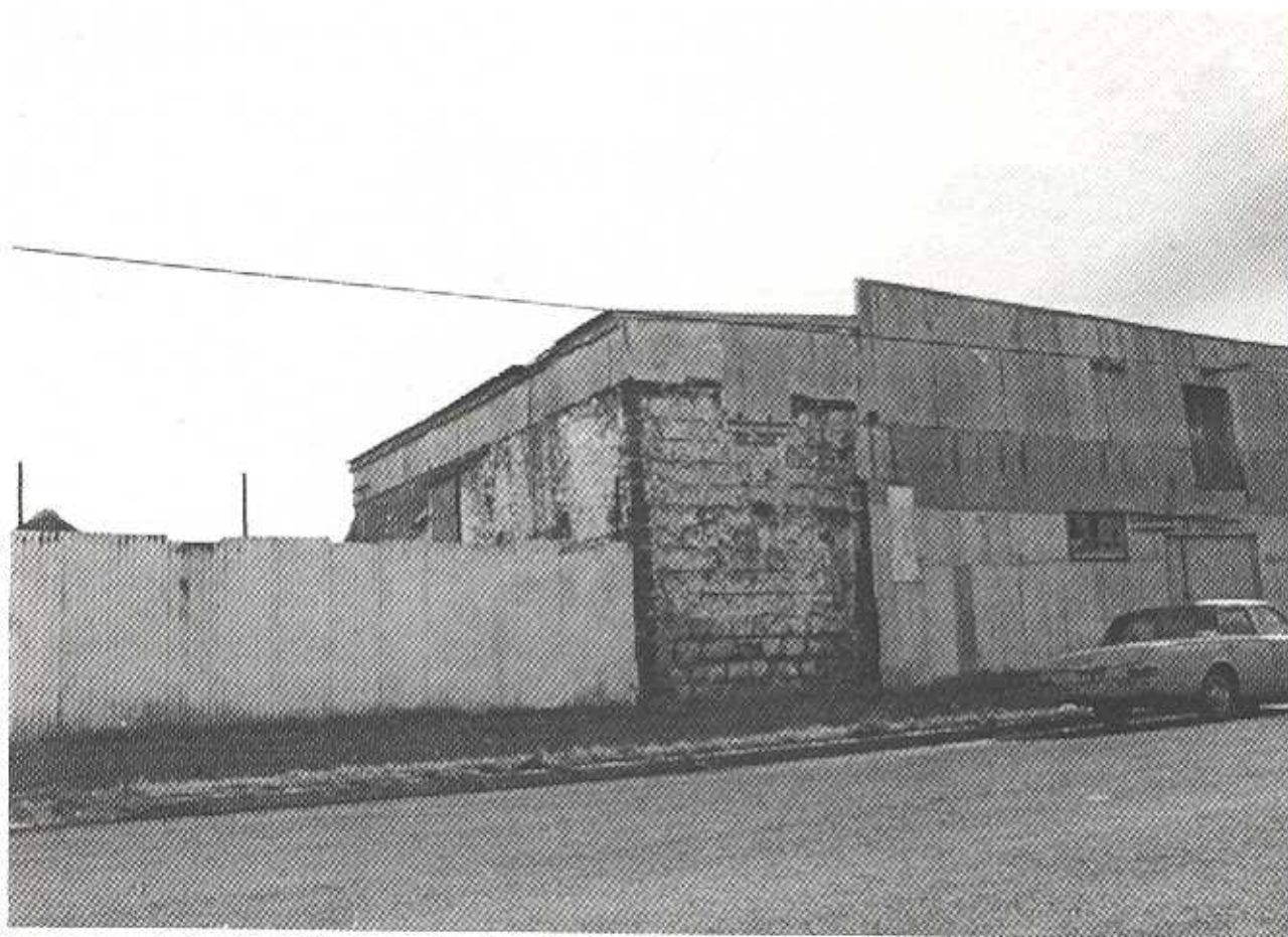
Basalt rubble possible engine room, now minus roof and timber framed store once attached on the north.
