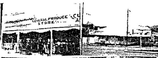
This important corner buildings is one of the earliest commercial buildings surviving in Buninyong, and dates from the early 1850's. The principal facade is constructed of brick with a parapet. A timber facade faces Warrenheip Street, and the structures are linked by a timber post supported verandah. A decorative timber valence completed the verandah and its reinstatement is recommended.
