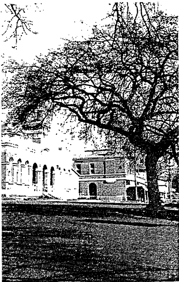
VIEW OF THE TOWN HALL FROM LEAKMOUTH STREET.
