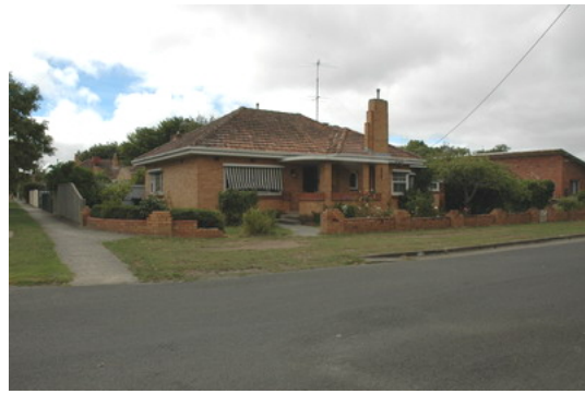
Photo 3.02: Dwelling, 14 Lindisfarne Crescent. Also note early low solid brick front fence.
