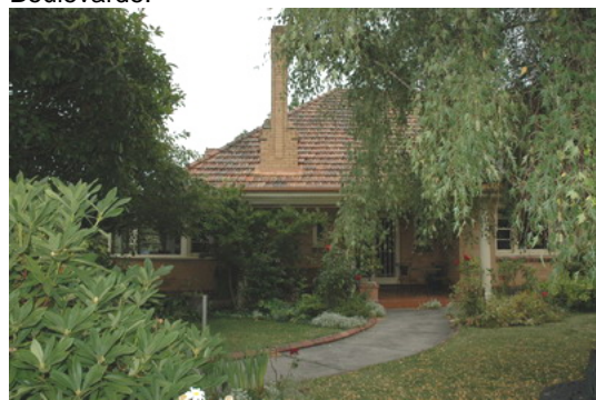
Photo 3.08: Waterfall style dwelling with curved bay (left side) and stepped chimney, 1 St. Aidan's Drive.
