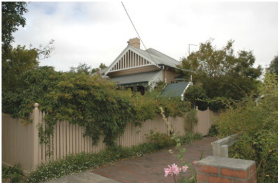
Photo 3.11: Edwardian dwelling (former Warden's Cottage, St. Aidan's College), 3 St. Aidan's Drive.
