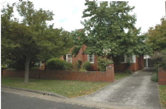
Photo 3.13: Early solid brick front fence, 7 St. Aidan's Drive.
