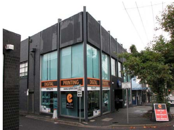
Figure 11 Caplan Motors Showroom, 194 St Kilda Road, St Kilda (1960)
