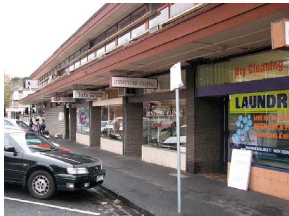
Figure 13 Detail of shopfronts to Carlisle House along the Westbury Street frontage
