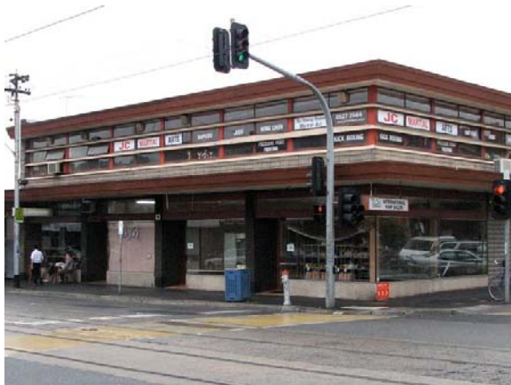
Figure 12 General view of Carlisle House at 320 Carlisle Street; Balaclava (1964)
