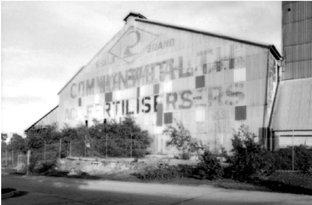
Figure 13 North end of Sheds 4, 5 & 6, showing 'Sickle Brand' and Cuming, Smith & Co. signage over-painted by Commonwealth Fertilisers after 1929. Source: Peter Bennetts, 2007.
