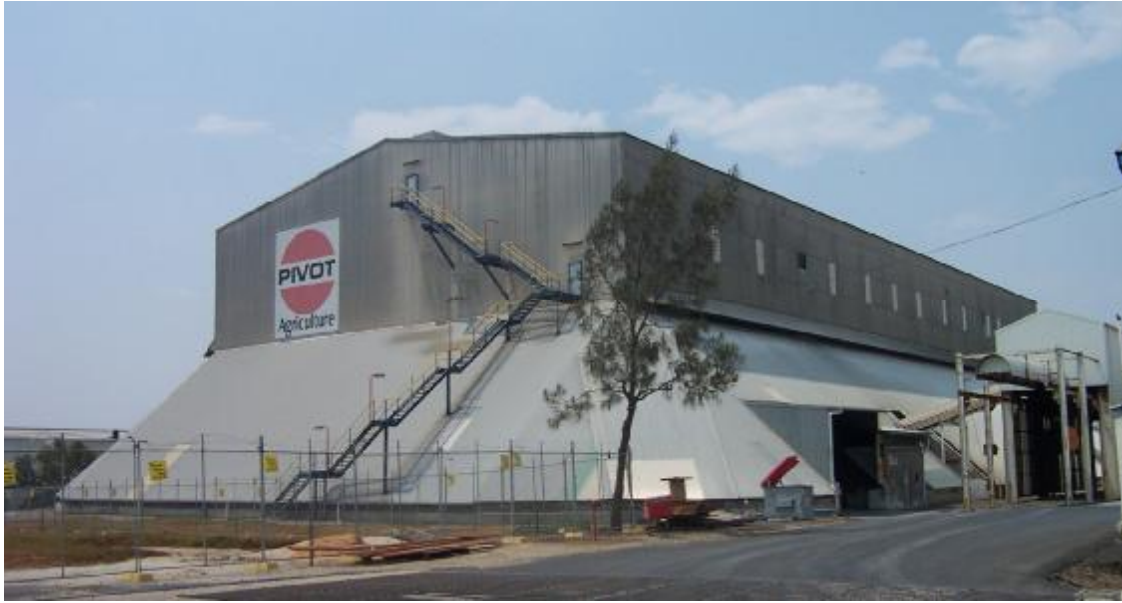
Figure 27 The enormous Shed no. 8, a landmark structure from the 1960s.
