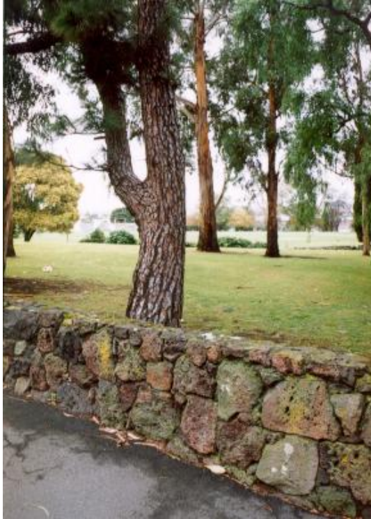
Fig 37 Extant stone wall to Yarraville Gardens/Hanmer Reserve along Hyde Street (built 1930s), show traditional construction, with broad base tapering to top, raked joints and capping row. Originally completed with a steel post and mesh fence above. Notice also the relationship of wall to conifer behind, for a strong textured theme (photograph Jill Orr-Young, 2000)
