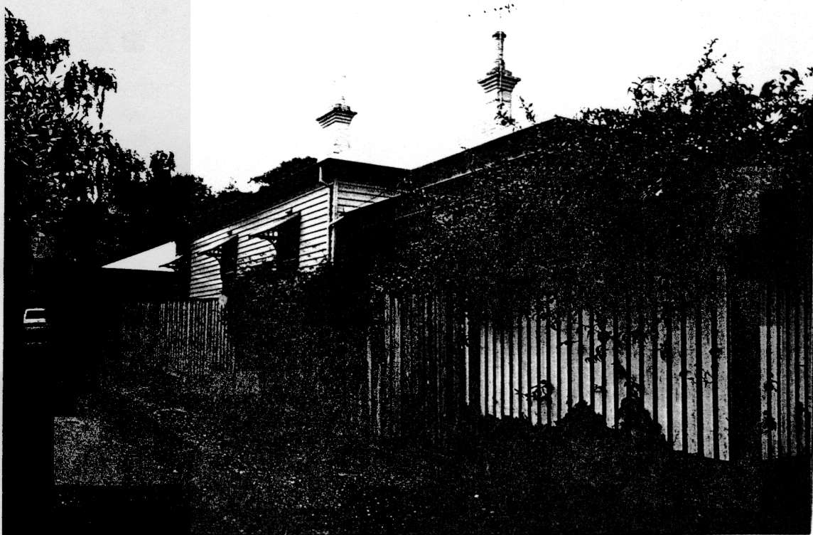
CHIMNEY POT 30 PLEASANT STREET RP. NTS. 8.2.97.
